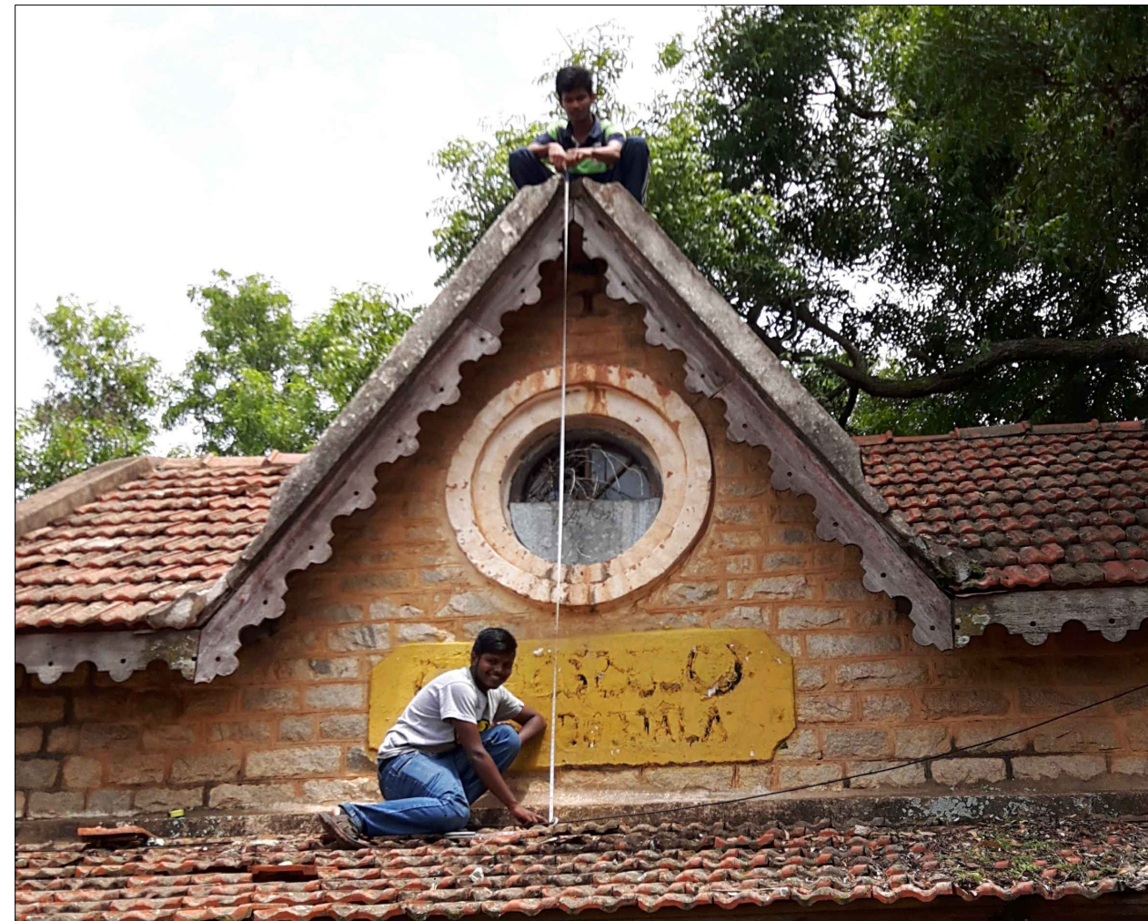
(Source: Photo Taken by Ar. Sharan Desai)
